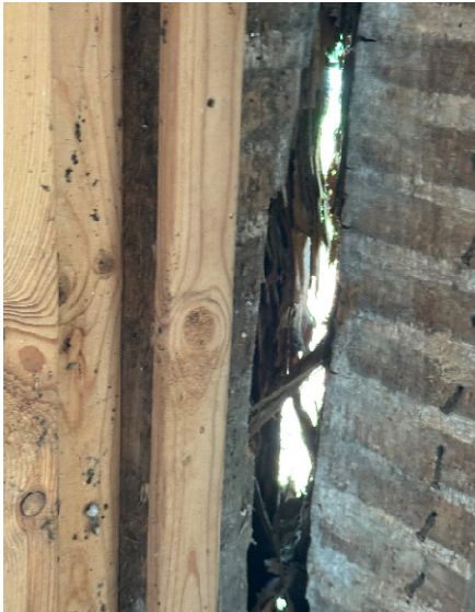
Photo 1: Termite Damaged 4x4 Post
