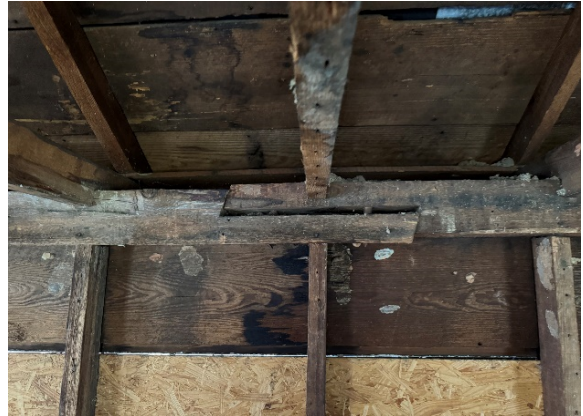
Photo 6: Differential Building Settlement
