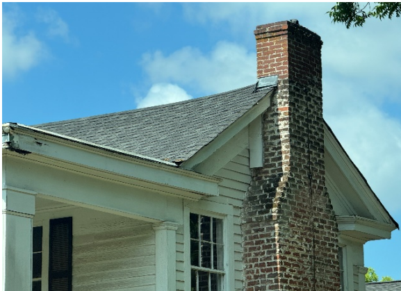
Photo 7: Differential Building Settlement
