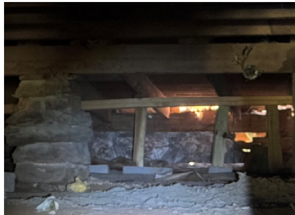
Photo 15: Retrofit Concrete Blocks Bearing on the Soil
