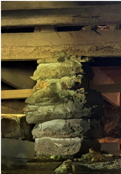
Photo 11: Stone with Mortar Foundation
