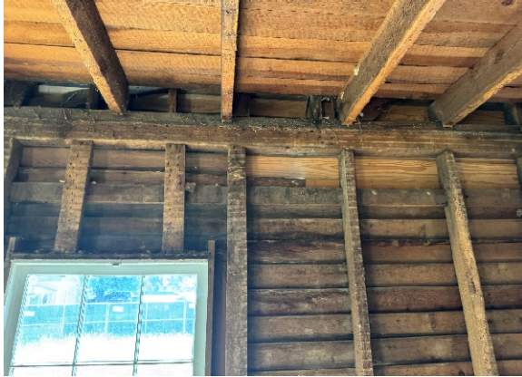
Photo 9: Differential Building Settlement
