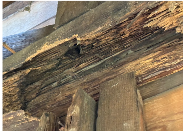
Photo 2: Rotten 4x8 Beams
