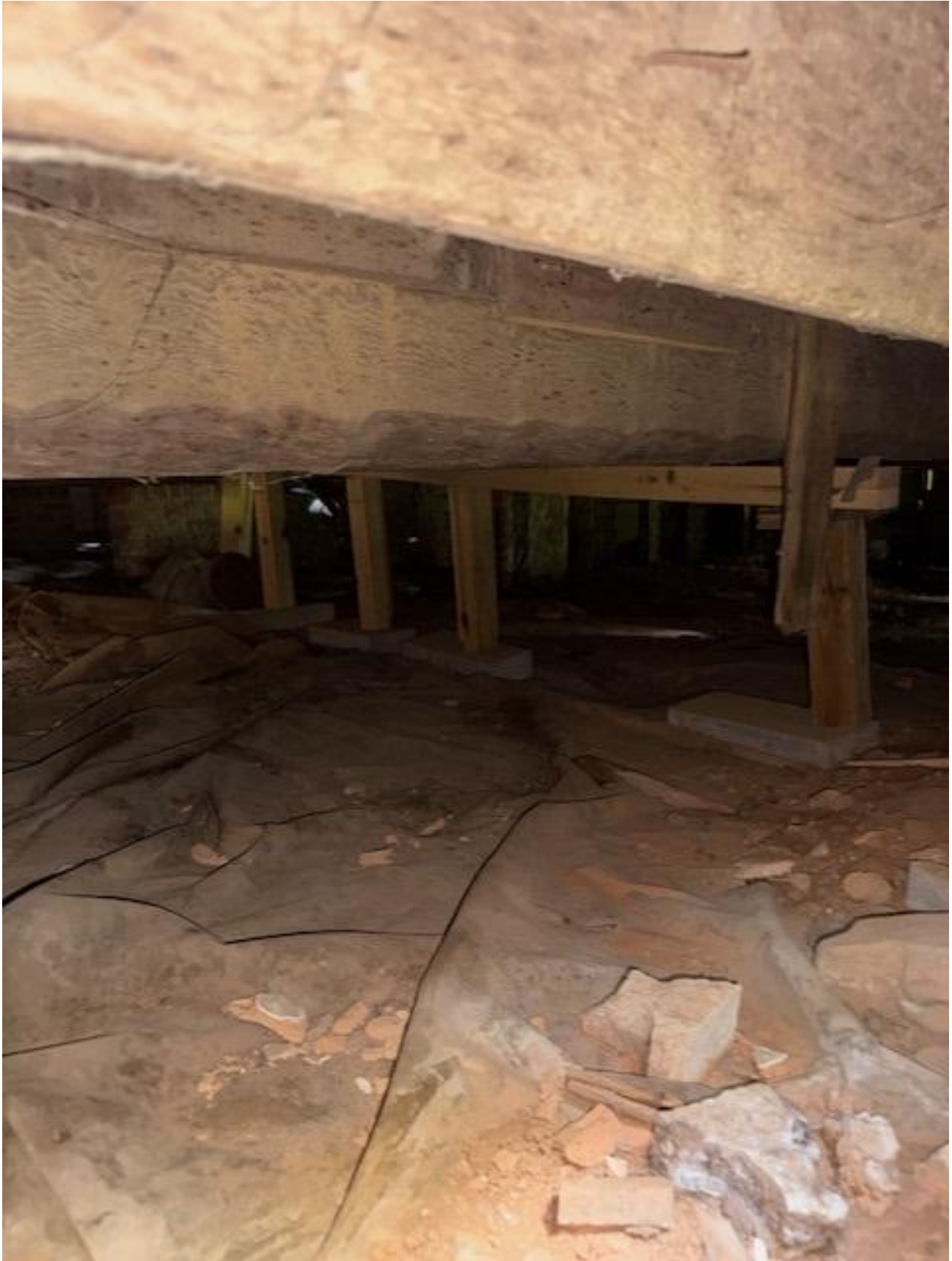
Figure 8. Foundational supports below the historic portion of the existing structure, some modern reinforcements appear to be present (photo from Staff)
