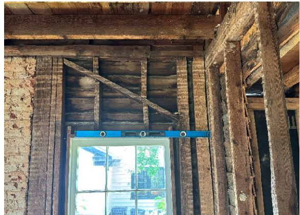
Photo 8: Differential Building Settlement
