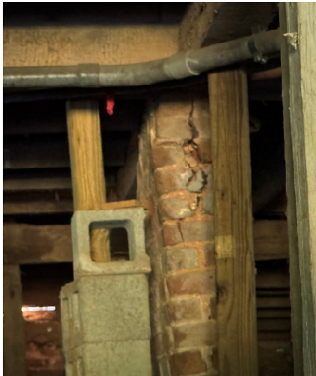
Photo 13: Brick Pier with Significant Crack
